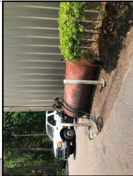
23 An approximate 250-gallon diesel fuel AST observed at Carolina Contractors (30 Hunter Road).
